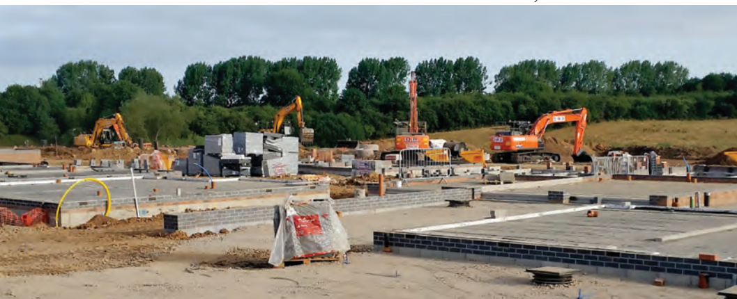
Structural board thermal floor system installation on-site.
