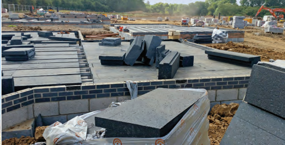
Lower Bardon – foundations, plot one.
