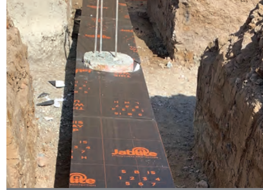
Ground heave protection installed on-site in Harrow.
